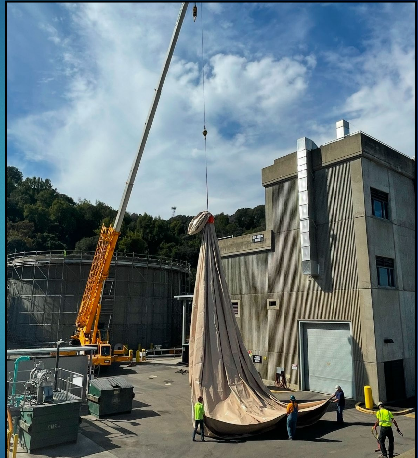
Digester Membrane Replacement
