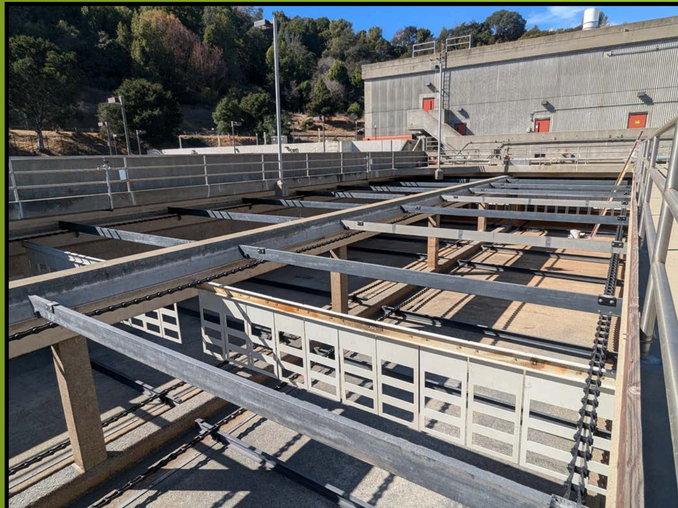
Flow Optimization Baffles Increase Organics Capture
